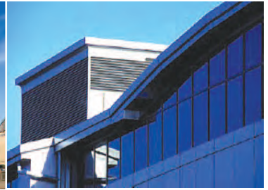
Bridge View Petrofac, Scottish Ministers
